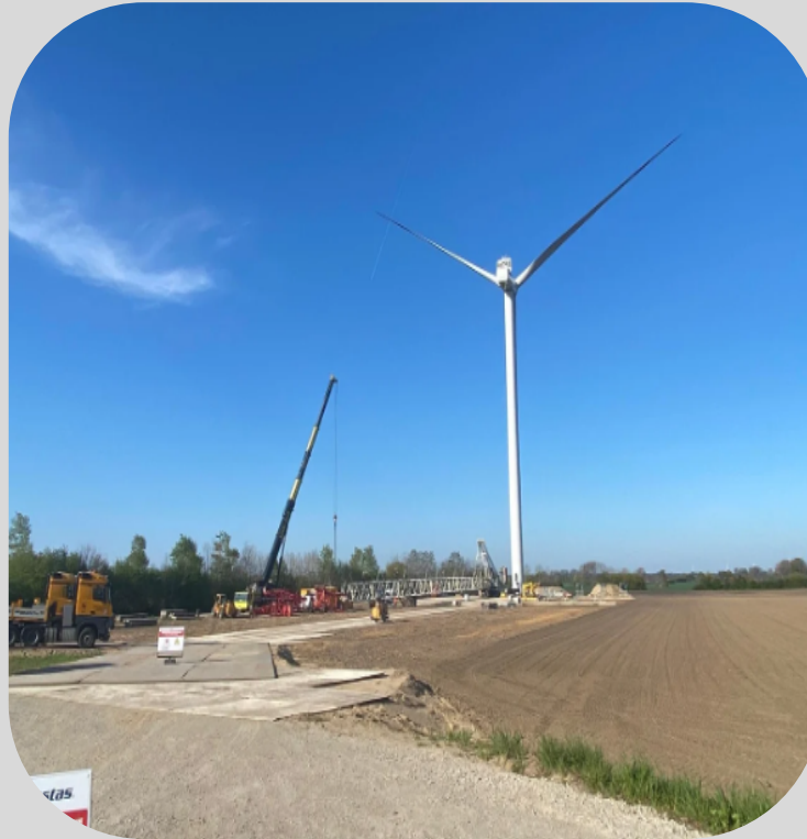
Figure 1. Construction of Windpark Grube
