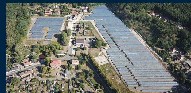
Aerial of Solar PV in Friedrichshain, ground mounted: operational
